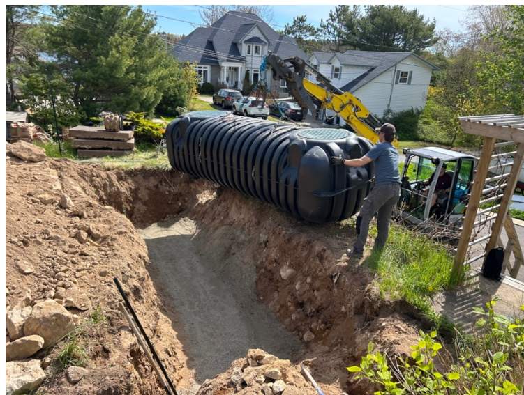
Figure 2: Installing a cistern
